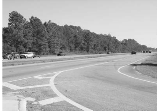
Figure 1. Example of Maneuver 2A: Improved intersection with higher speed roads with right-turn channelization at an intersection; an acceleration lane is present and sloping curbs are painted.
