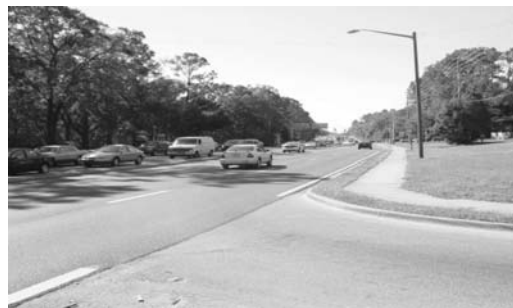
Figure 2. Example of Maneuver 2B: Unimproved intersection with higher speed roads with right-turn channelization at an intersection but with no acceleration lane; curbs are not painted.
